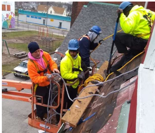
Seagate Roofing installed a new roof in March 2020.
