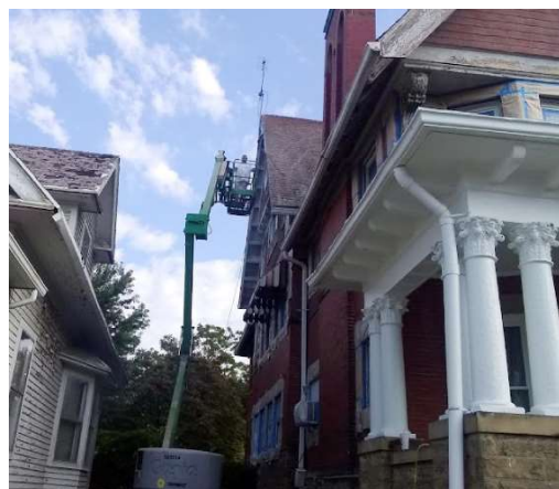
Chittum Painting began Padua Center's face lift in August 2019.
