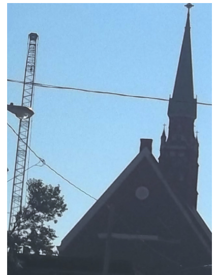
A large crane looms over St. Anthony Church. The crane and other equipment arrived on June 1, 2018.
